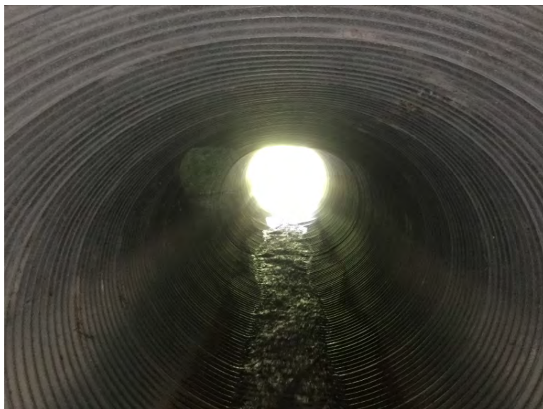
Damage to roof at midspan
